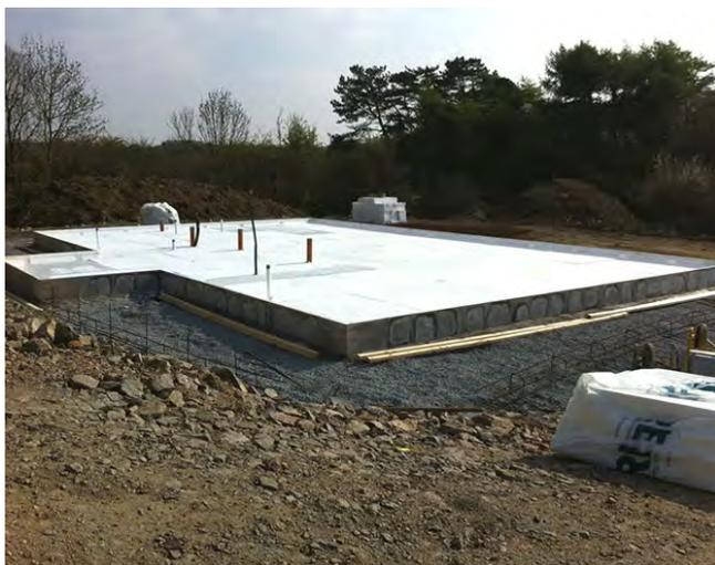
This load bearing insulated foundation system helps eliminate thermal bridging from foundations.
