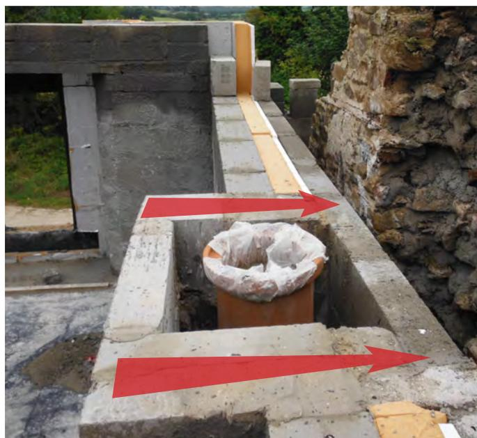
The arrows in this photograph show where a thermal bridge has been formed by the chimney structure which passes right through the insulation layer.
