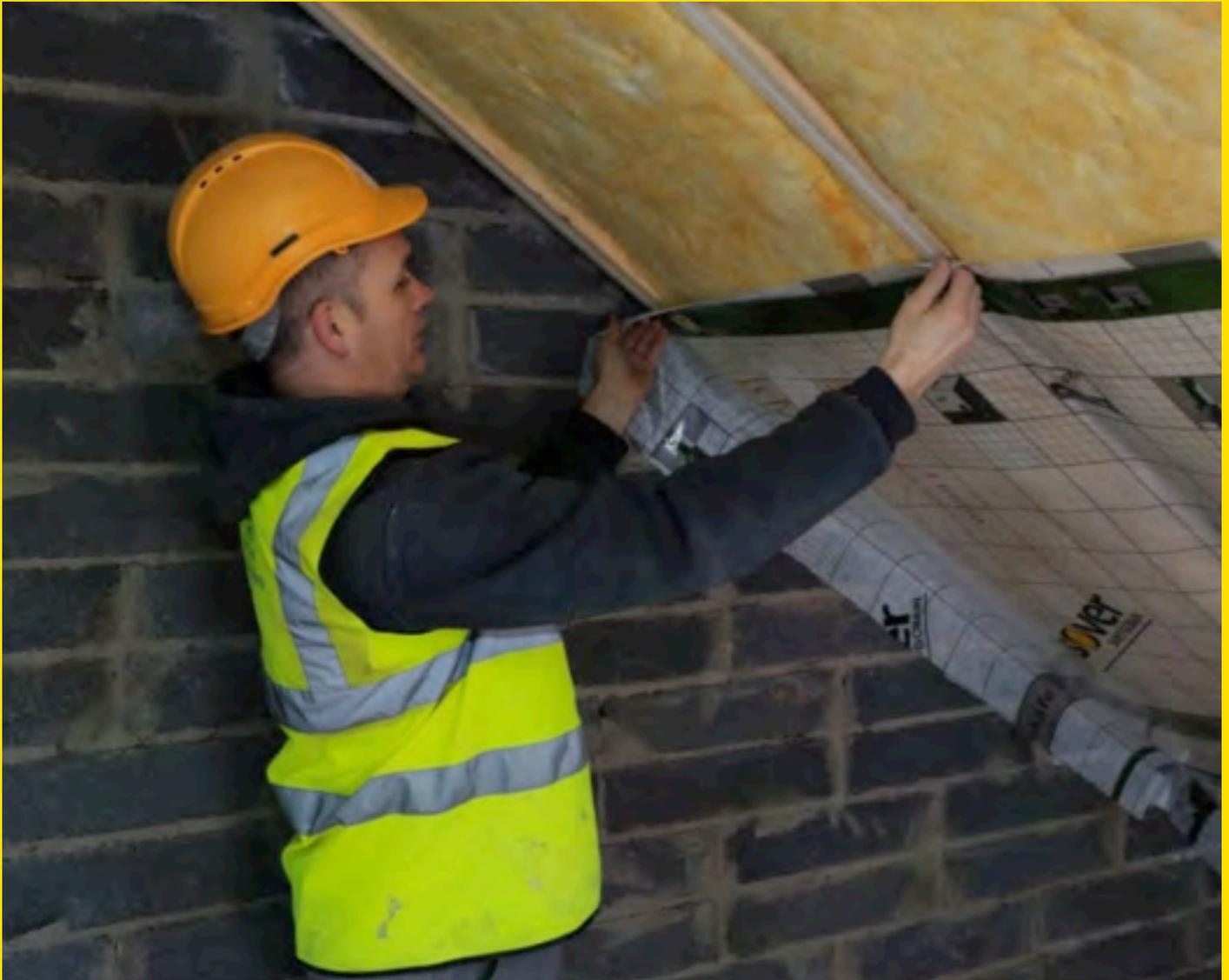
*Vapour Barrier applied carefully to underside of Rafters in attic to prevent moisture getting in. This also requires a ventilation space above the insulation to avoid interstitial condensation.
