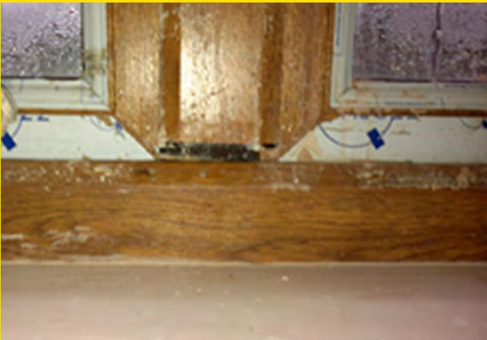
Surface condensation on windows due to heat loss through the windows and the incorrect levels of ventilation
